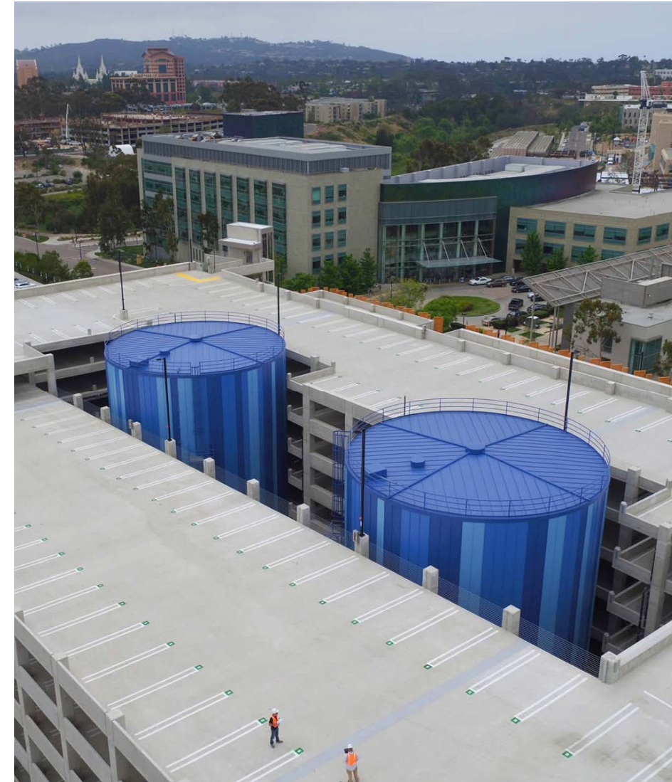
Thermal Storage Tanks (TES)
