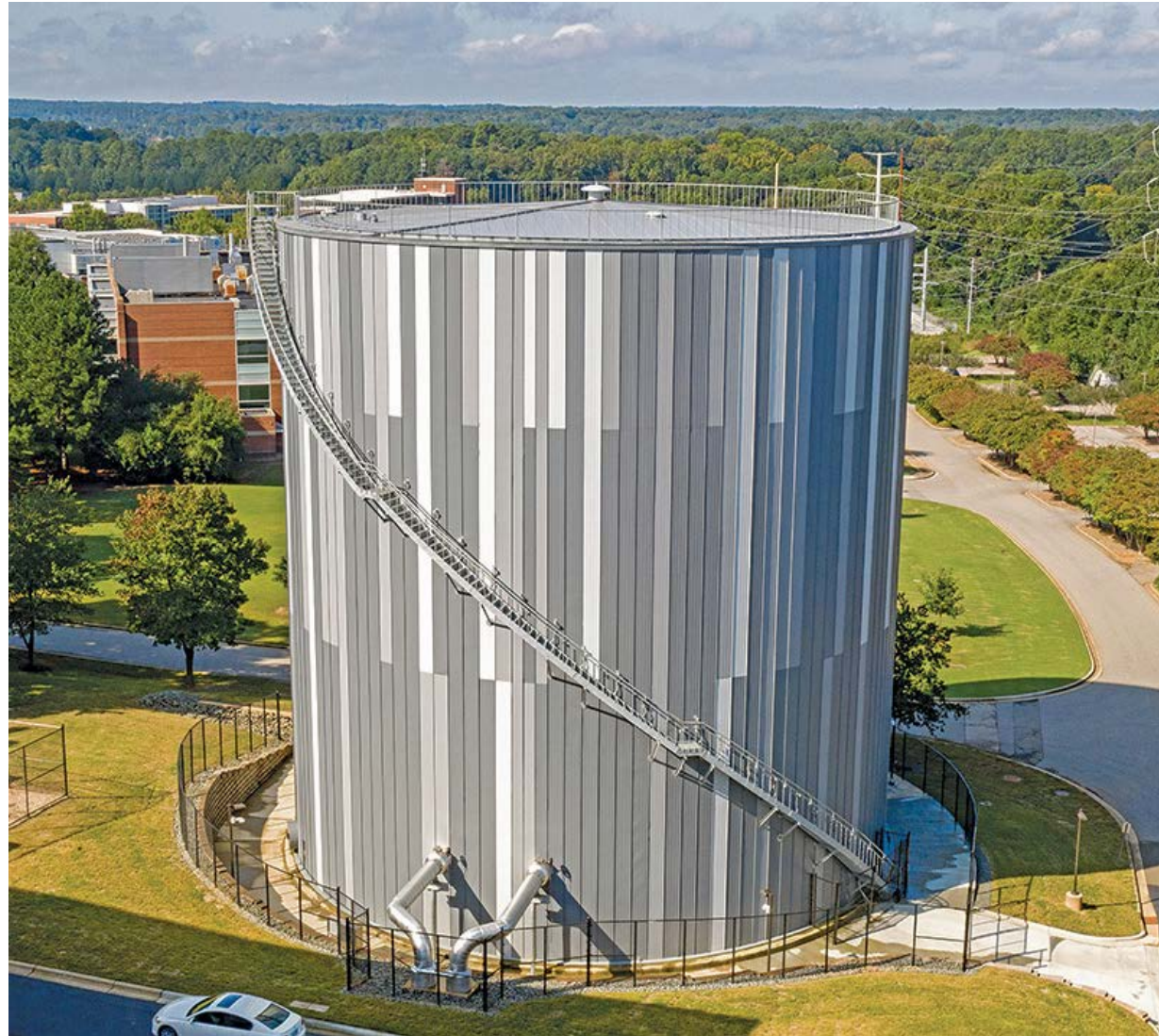
Thermal Storage Tanks (TES)
